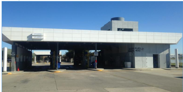
Fueling station at SamTrans North Base Facility.
