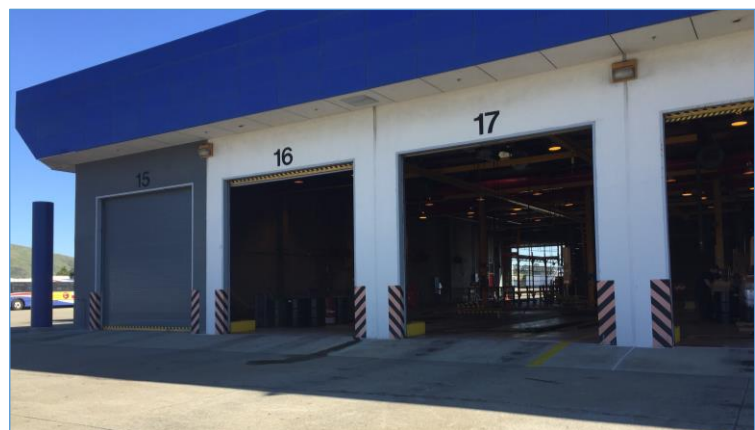
Auto shop at the SamTrans North Base Facility.
