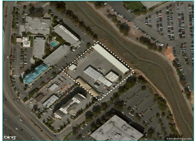
Mid-Level Scenario: Asset under 0 to 5 feet of water.
