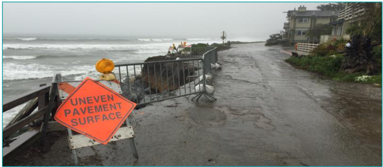
Eroded segment of Mirada Rd with temporary riprap protection.
