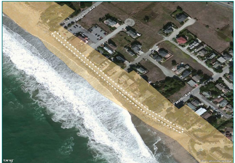
Erosion Analysis: Site is entirely in future erosion area.
