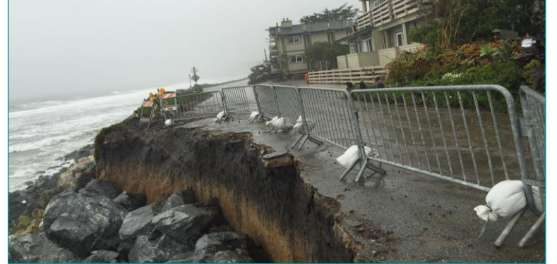
Eroded segment of Mirada Rd with temporary riprap protection.
