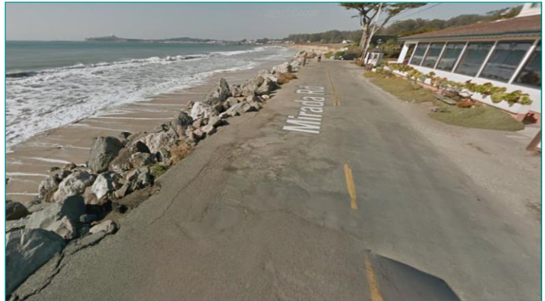
Google Street View showing poor but functional maintenance.
