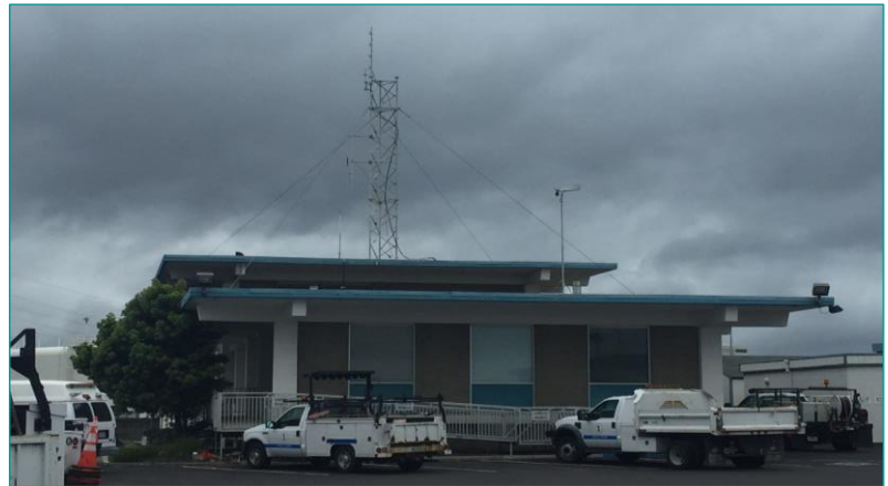
Communication tower with emergency broadcast function.
