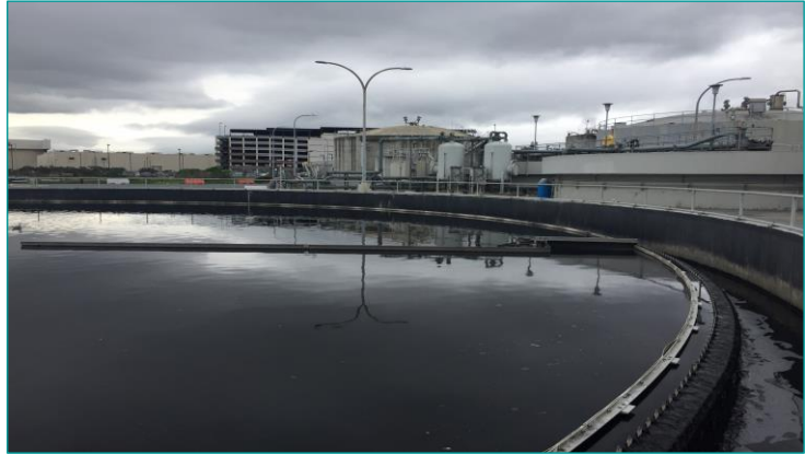
Secondary clarifier, looking south.
