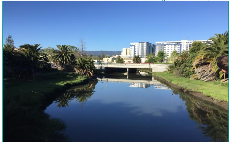
Redwood Creek can overtop and cause flooding at the facility.
