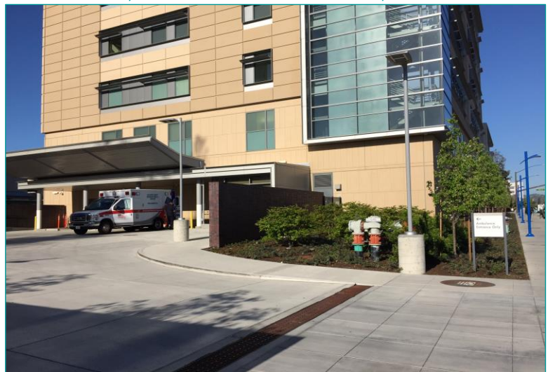
ED entranceway for ambulance is a critical component of asset.
