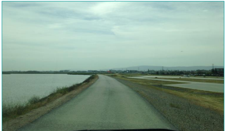
Levee system that reduces flooding at San Carlos Airport.
