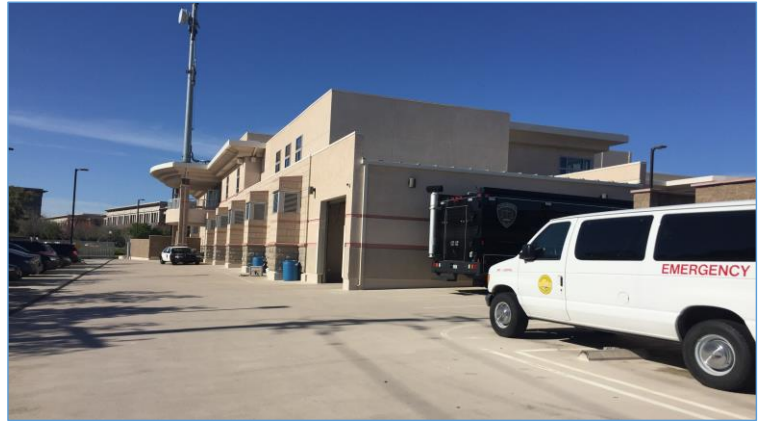
Police department station and specialized vehicles.
