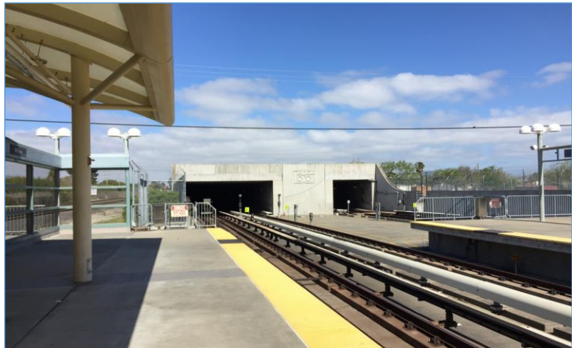
Entrance to BART tunnel at Millbrae Intermodal Station.
