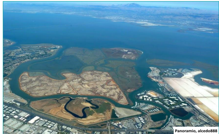
Aerial view of Highway 101 section adjacent to wetlands.
