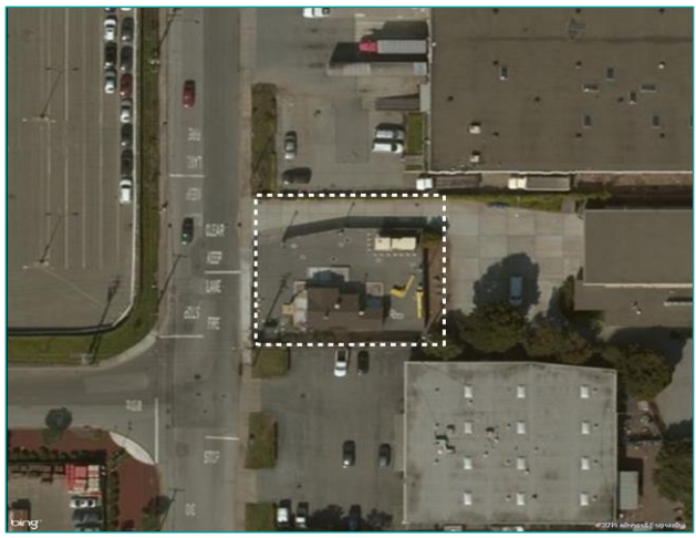
Mid-Level Scenario: Asset flooded 1-4 feet deep.
