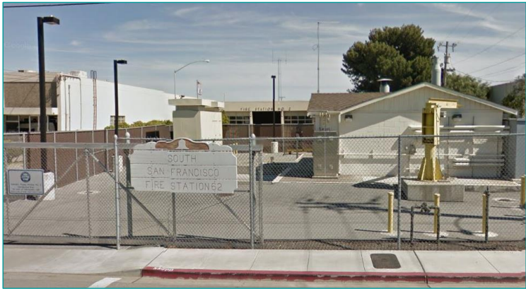
Google Street View of Pump Station Number 4.
